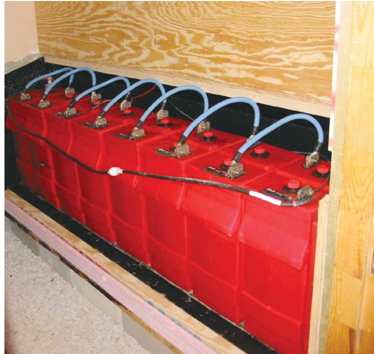
This battery box, with a removable front, makes future battery replacement easier.
