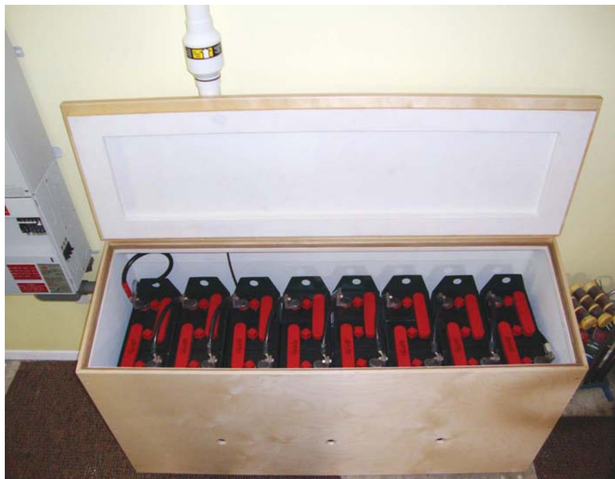
A peek inside this battery enclosure shows a clean installation, with ample room for the battery cases and interconnects.
