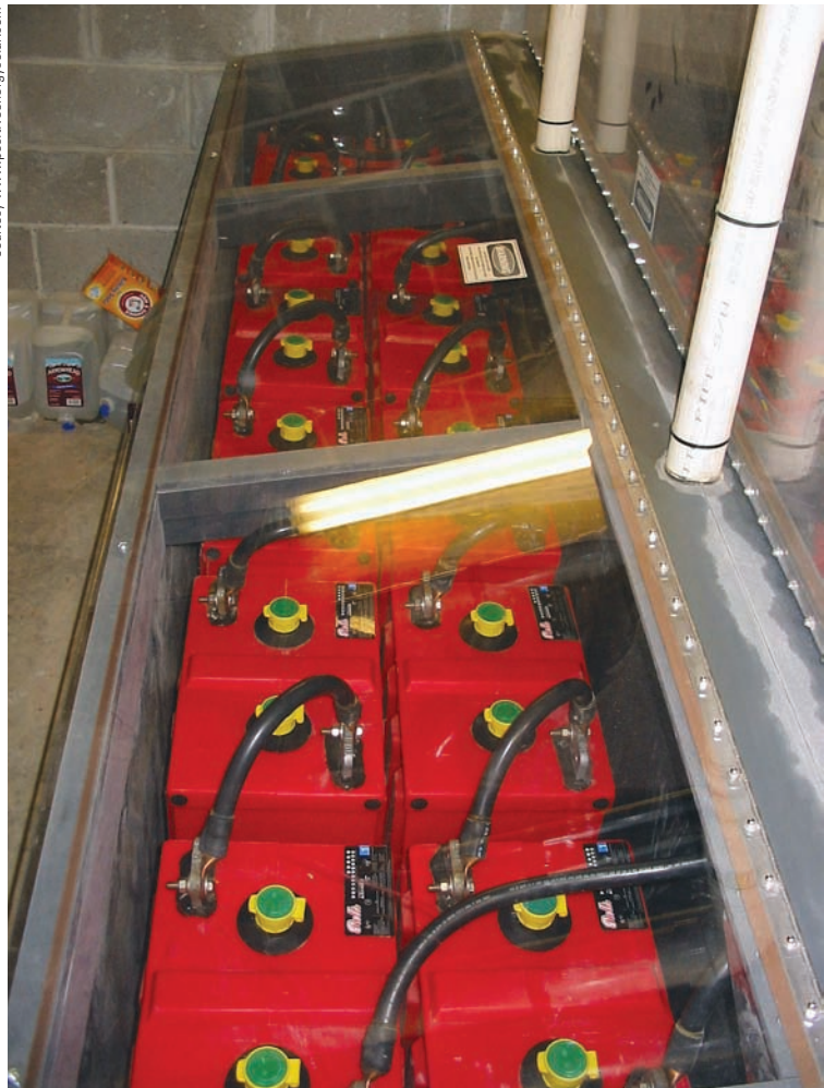
A well-constructed, site-built battery enclosure.
